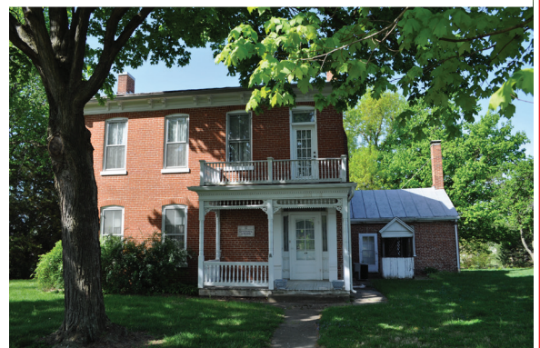
The Bellefontaine House is located at 709 South Church Street in Waterloo.
